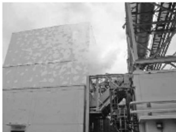
Fig. 1 Steam coming out of a blow-out panel opening at the Fukushima Dai-ichi Unit 2 Reactor Building on March 15, 2011
